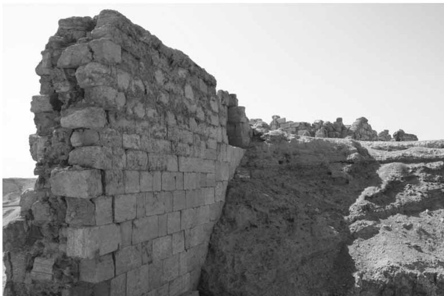
Figure 1: The northern extremity of the citadel wall looking south. Notice the weathering on the upper region compared with the comparatively good preservation of the more recently exposed area of wall (Joshua Bryant).
