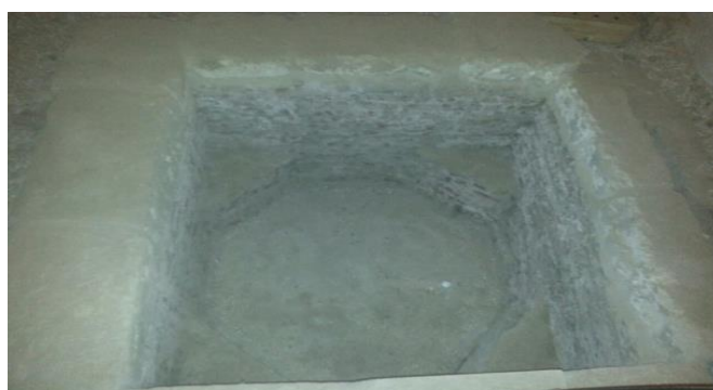
Fig. 13 - The octagonal Maghtas , inscribed in a square in the palace of Saint Helena in the monastery of Saint Bishay, stone, 1.50 m deep. (©Author's photography)
