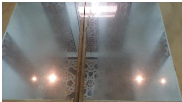
Fig. 11 - The rectangular Maghtas covered with marble in the Abu Sergah church, black and red marble, 1.40 m deep, 2.60 x 1.7 m length and width. (©Author's photography)
