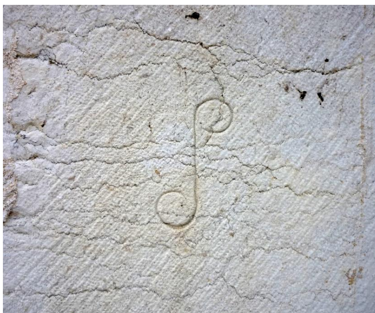
Fig. 7 – Example of stonemasons' marks and surface treatment, north of the Church of S. Maria Maior (photo: Dorothee Heinzelmann, 2011).
