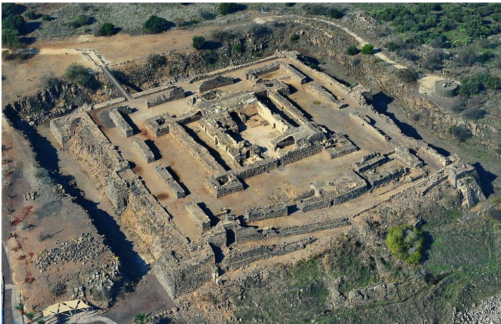
Fig. 4 – Aerial view of Belvoir Castle (Source: https://en.wikipedia.org/wiki/Belvoir_Castle_(Israel) ).
