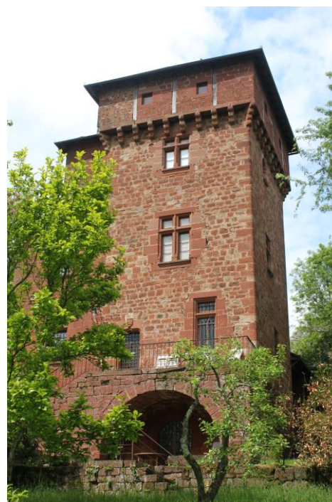
Fig. 2 - Tower of the house of Les Landes in Mouret (Aveyron) (©Y. Mattalia).
