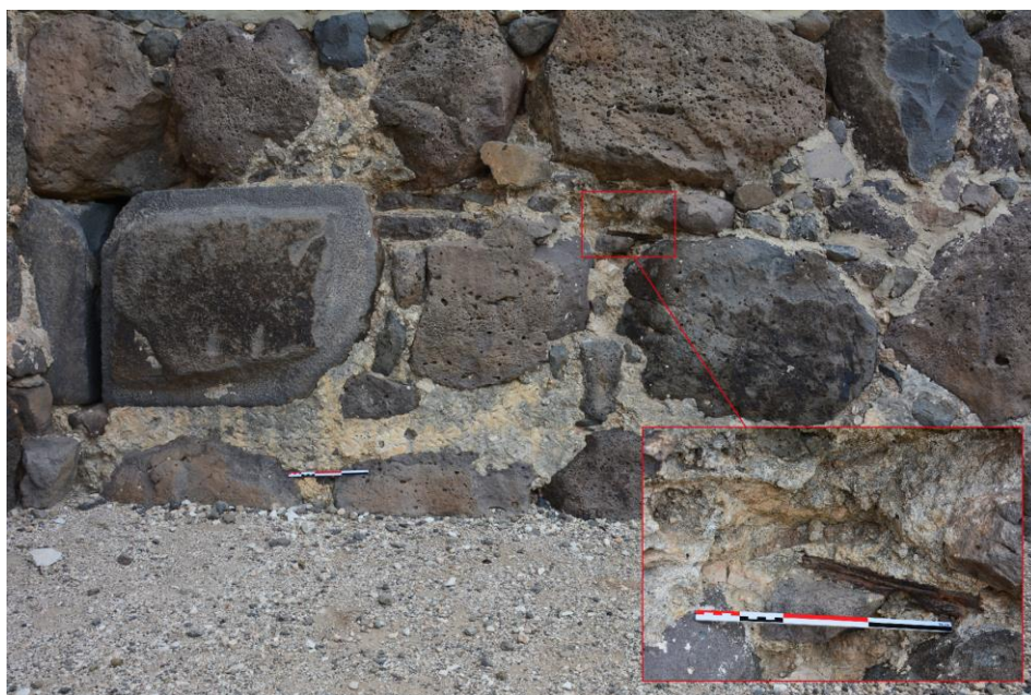
Fig. 5 – Iron staple between two blocks of basalt (© A. Baud).
